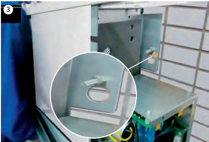
Tighten the expansion screws on each side.
