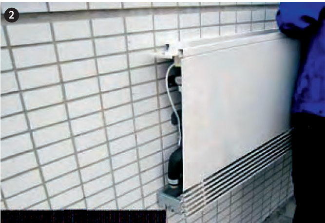
Secure the unit with metal expansion bolts.
