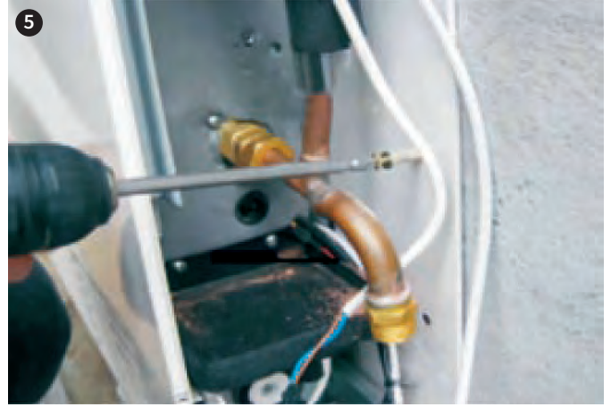
Secure the unit with screws.
