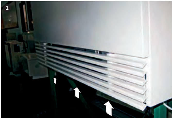
Press and pull to remove the air outlet grille.
