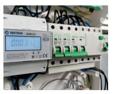
Electricity meter allows for monitoring the energy consumption of the heat pump.
